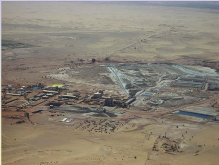
Aerial view of Areva's Somair mine
